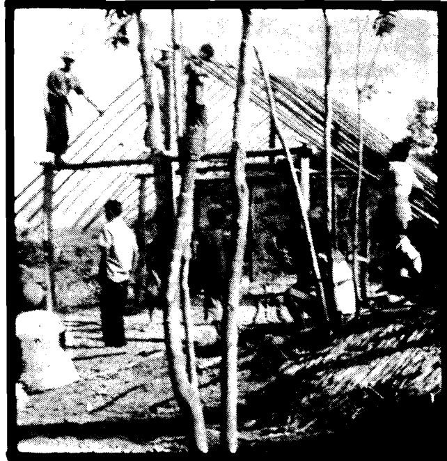
BELOW: This new structure will be made of bamboo and reeds in the traditional Lahu tribal style.
