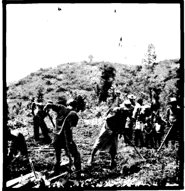
ABOVE: The men break and level the ground for their new church building in Burma.
